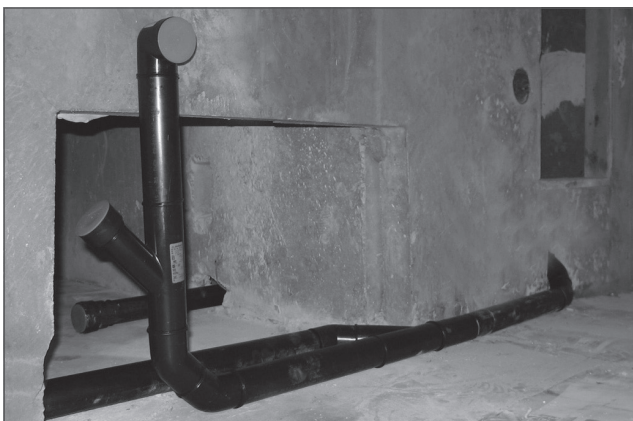
Illustration 9.2 Prefabricated pipe sections installed on site
