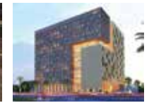
Hilton Garden Inn Hotel & Doubletree Suites, KSA (Wefatherm)
