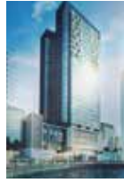
Crowne Plaza Dubai Marina, Dubai, UAE (Sanit)
