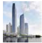
The Address Harbor Point, Dubai Creek, UAE (HDPE & dBlue)
