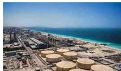
Jubail phase IV potable water plant, KSA (FIP)
