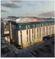
Aloft Hotel Garhoud, Dubai, UAE (dBlue & HDPE)
