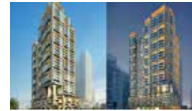
Al Wafra Tower - Reem Island, UAE (HDPE & Marley)
