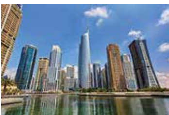
DMCC, UAE (Friatec)
