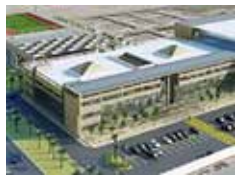
American International School Jeddah, KSA (Wefatherm)
