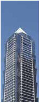
Al Batha Tower, Business Bay, UAE (Marley)
