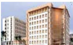
National Hospital Riyadh, KSA (Wefatherm)
